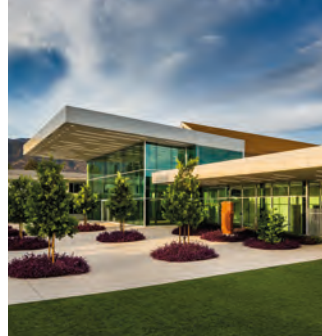
Above and top left: The new foyer features a dramatic roof with a cantilevered overhang Top right: The venue now seats 600, but a motorized roll drop can cut the space in half for more intimate productions Below: The sanctuary before its transformation into a performing arts center
